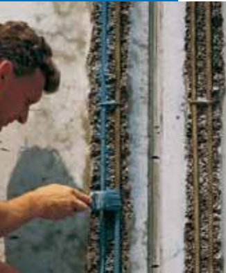
Application de Mapefer
