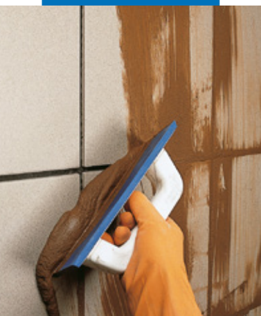
Grouting an external wall with a float
